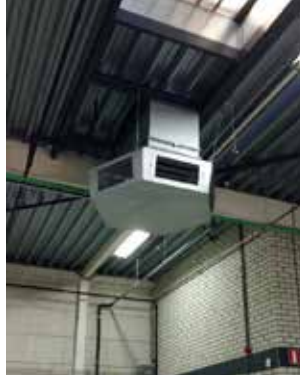
6-sided hexagonal air blowing plenum with horizontal louvers
